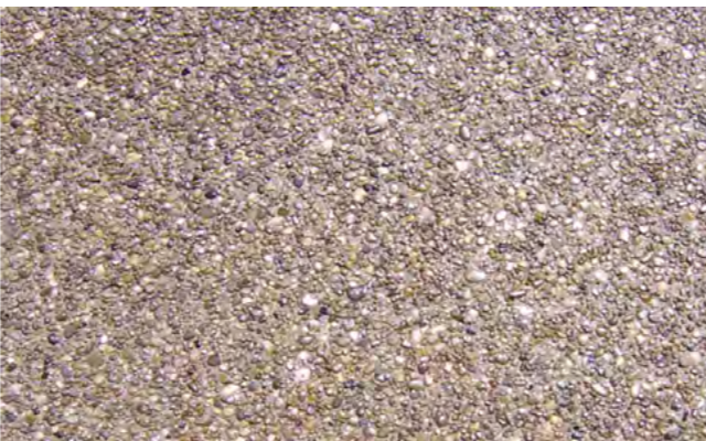
concrete with exposed aggregate
