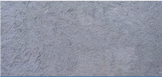
broomed finished concrete
