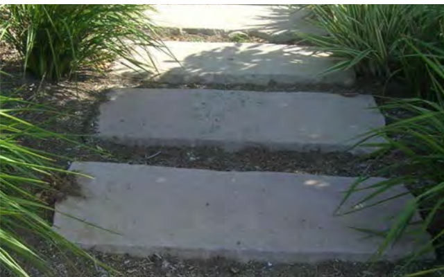
concrete paving stones
